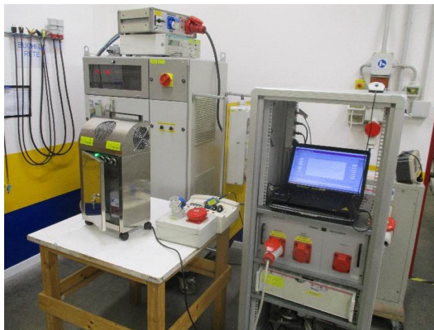
Measurement of voltage fluctuating and flicker
